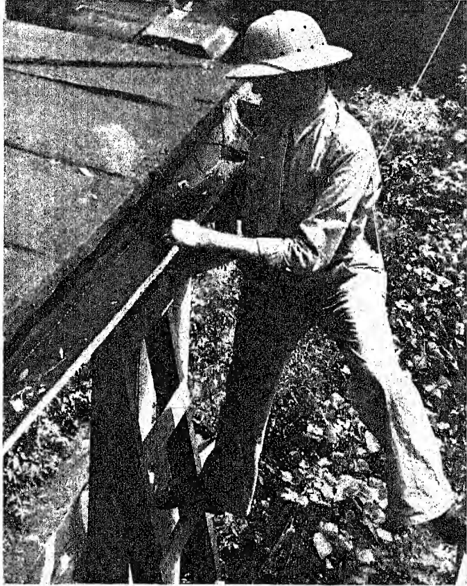
Figure 70. Cleaning a clogged roof gutter, to prevent the breeding of Aedes aegypti and other domestic mosquitoes
